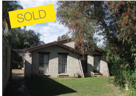
8 Nailon Place, Mona Vale
