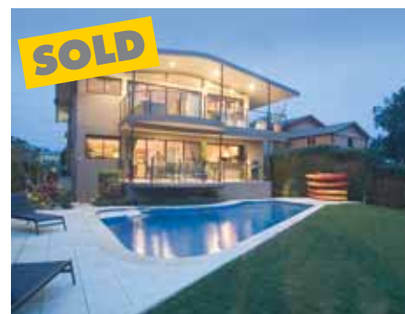
105 Wimbledon Ave, North Narrabeen
